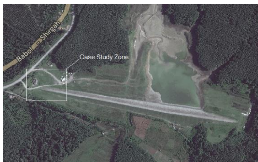
Fig.2. Sonboleroud dam satellite view
